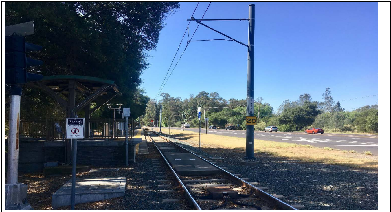
Viewpoint 4. Looking south at the Glenn Station. Trees, shade structures, and the concrete boarding platform, along with the light rail tracks and the OCS, and the proposed location of the new boarding platform, are visible in the foreground and middleground. Folsom Boulevard and trees in the Folsom Lake SRA are visible in the foreground, middleground, and background.
